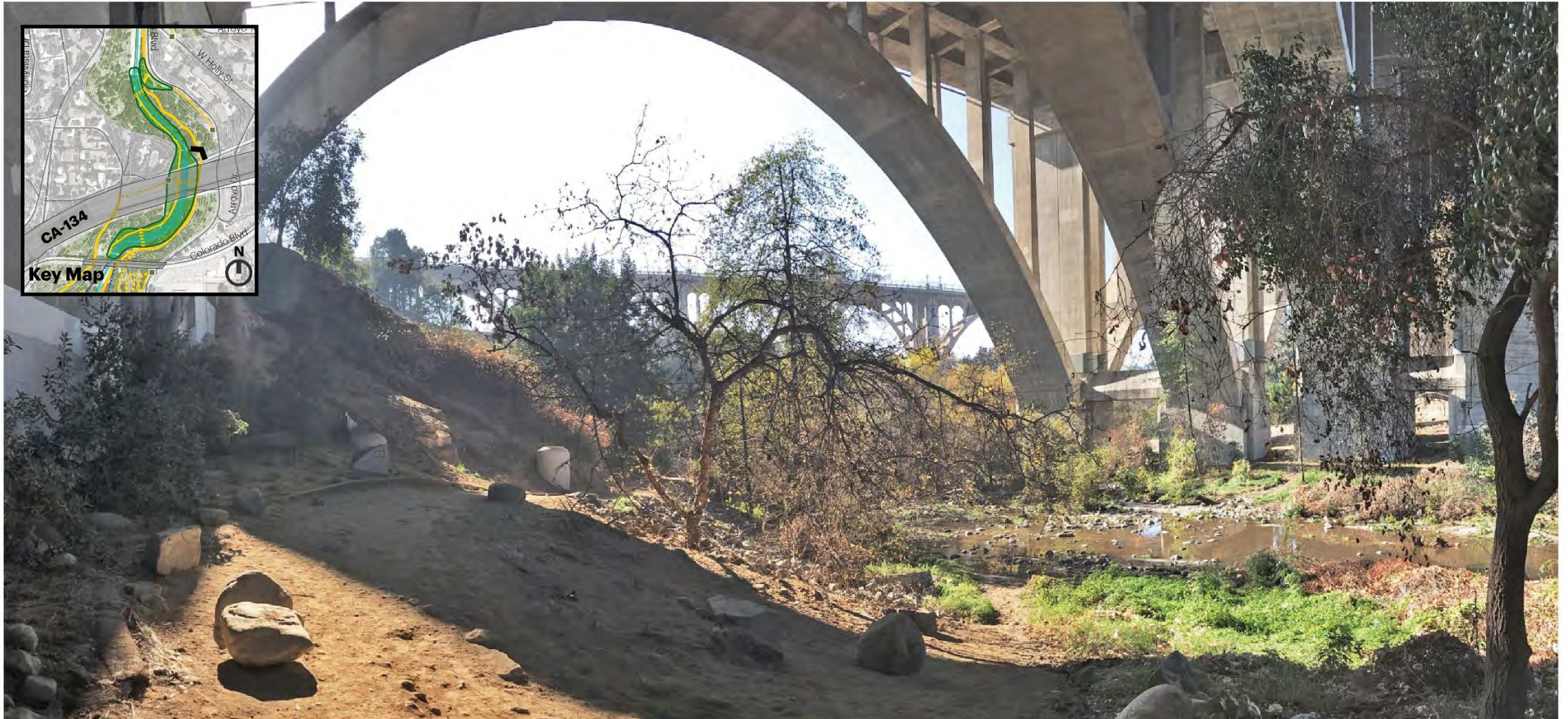
Existing conditions under CA-134 overpass
