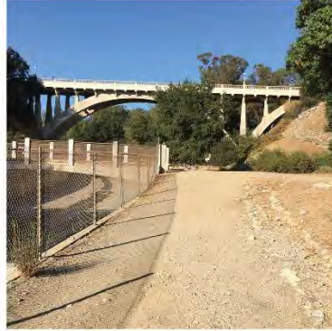
Trail along Lower Arroyo Channel
