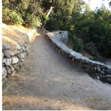
Feeder trail condition
