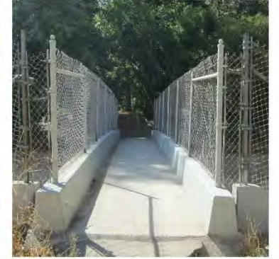
Bridge to be improved
