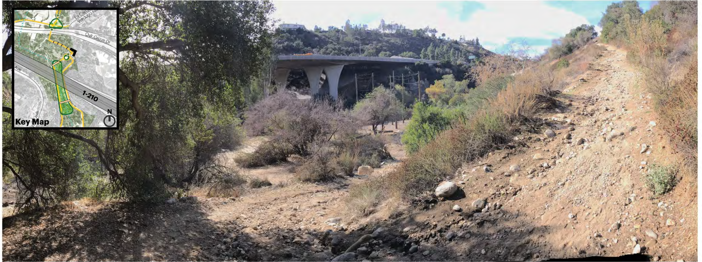
Existing conditions at base of switch back trail
